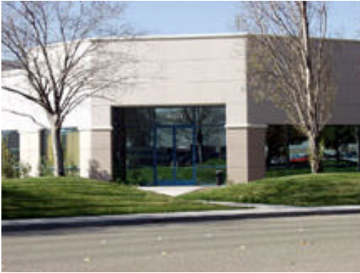
ACCESS Systems America (US, Fremont)
